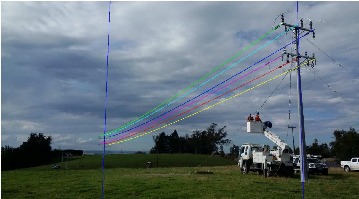
Figure 2: Surveyed conductor positions captured by LineSmarts
